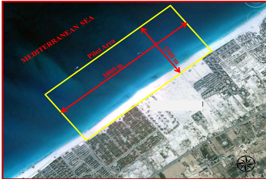
Fig. 2. Satellite image of the project area along the North-West coast of Alexandria
