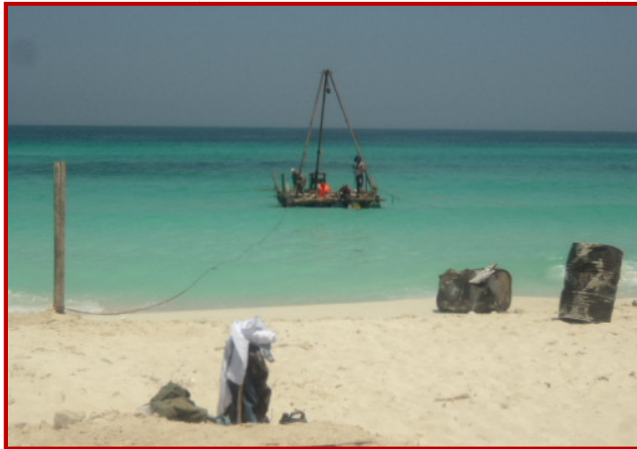
Fig. 4. The bore holes implementation in the site
