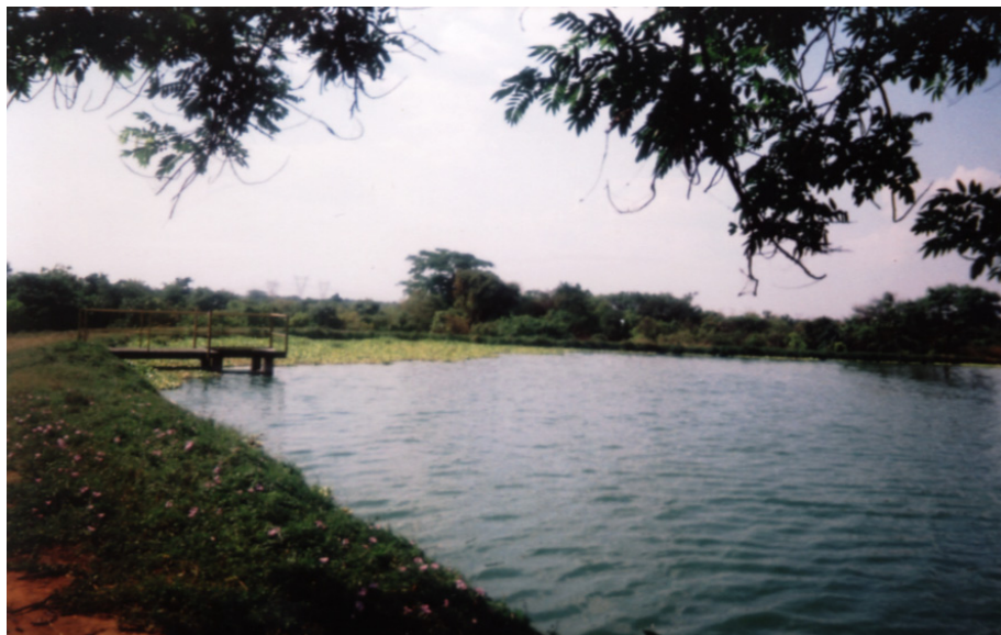
Figure 8. Kantanshi Sewerage Stabilization Pond in Mufulira
