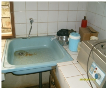
Fig. 2. Sinks through which effluents are drained in the laboratory of the hospital of Abomey-Calavi
