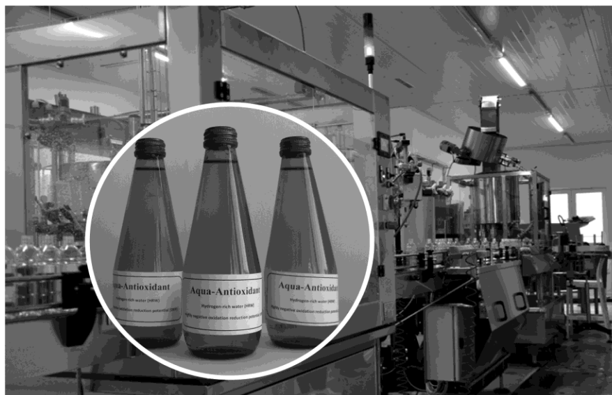
Fig. 3. Fragment of the installation - a bottling line for filling bottles
