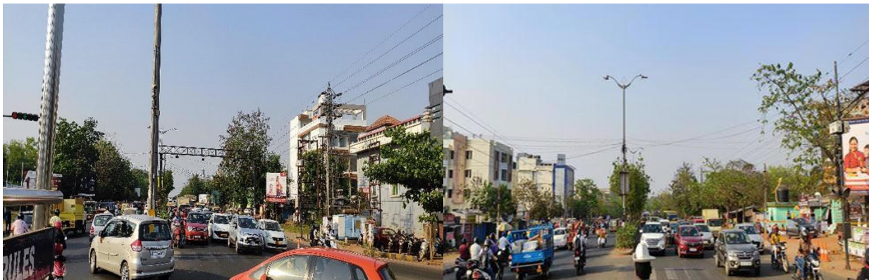
Fig 1 (a) Existing Condition of Kalinga Square Fig 1(b): Existing Condition of Damana square
