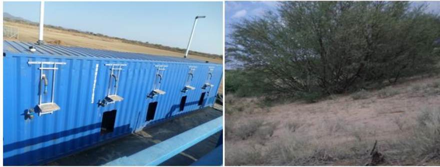
Fig. 9. Effluent treatment bio-box and vegetation irrigated by treated waste water
