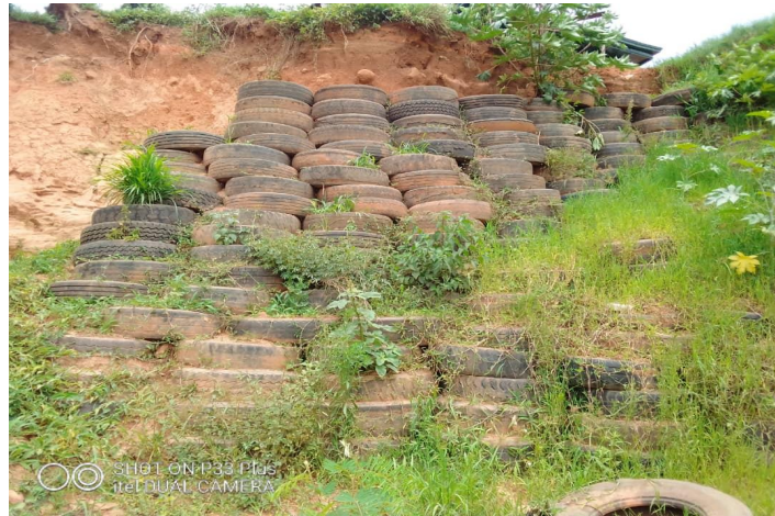
Fig. 3. Embankment constructed by the use of tyres Source: Fieldwork 2020
