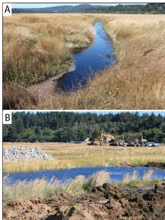
Figure 14. Constructed channels in the Ni-les'tun Unit
