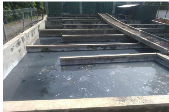
Fig. 5. Tofu Waste Treatment Plant, Central Lamper Village, Semarang-Indonesia
