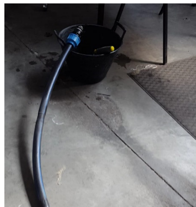
Figure 2. “Sausage effect” during the pressurization hydraulic test.
